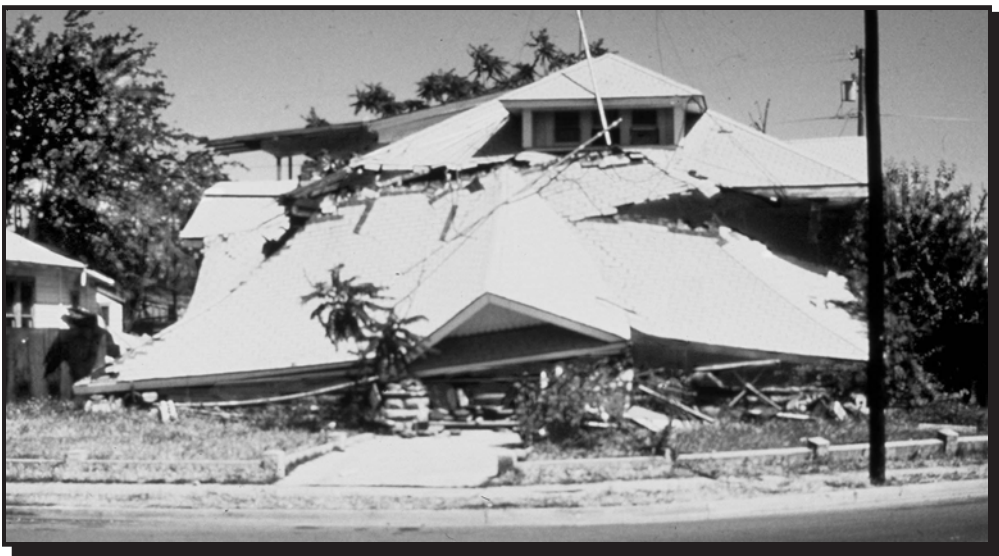
Additional damage from aftershocks
