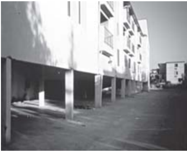
Figure 30 —Apartments with tuck-under parking like this can collapse. This building is leaning but did not collapse in the 1994 Northridge earthquake.
