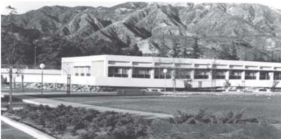
After the Earthquake
