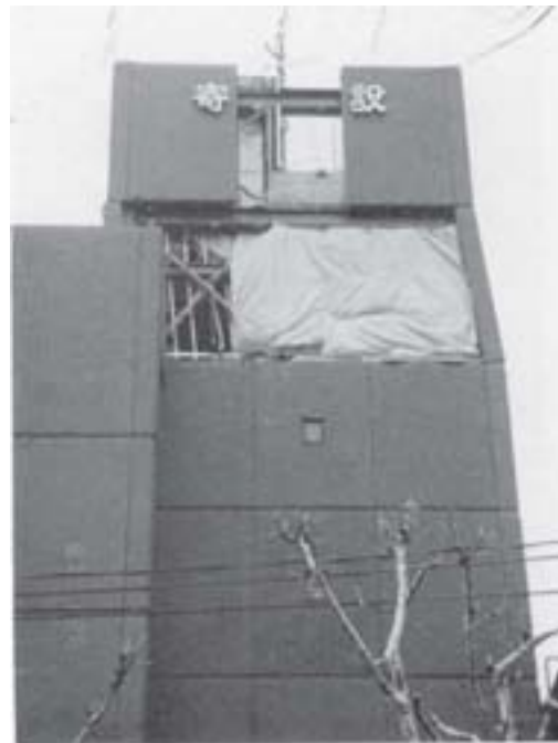
Figure 29 —A six-story steel braced frame building was damaged after the 1995 Kobe Earthquake in Japan. 4,000 to 8,000 small commercial buildings and 1,000 to 2,000 large commercial buildings were destroyed or severely damaged in that event.
